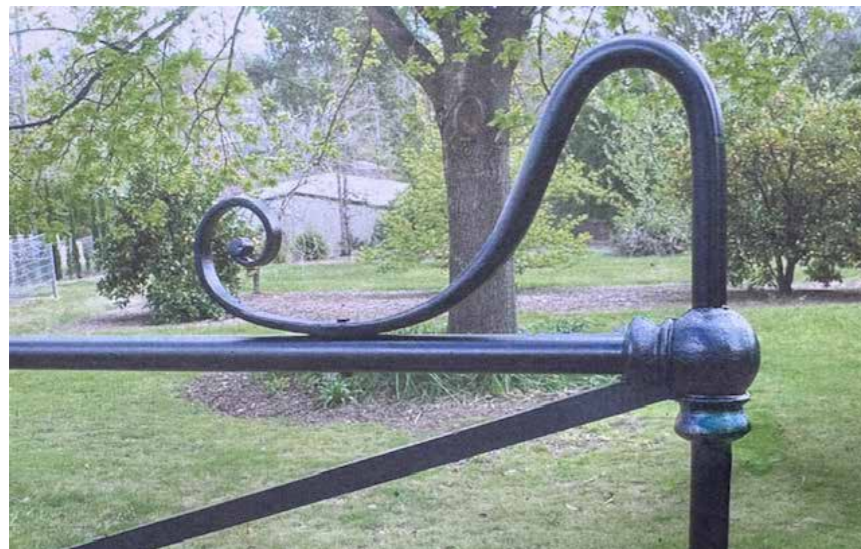
Hot-forged scroll detail with insitu aluminium alloy cast over and around full penetration fusion-welded frame.
