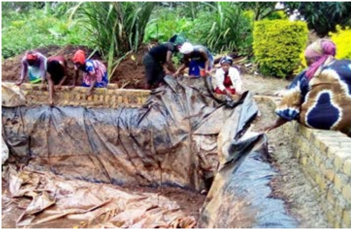
Water pit construction in Uganda SOURCE: St Jude
