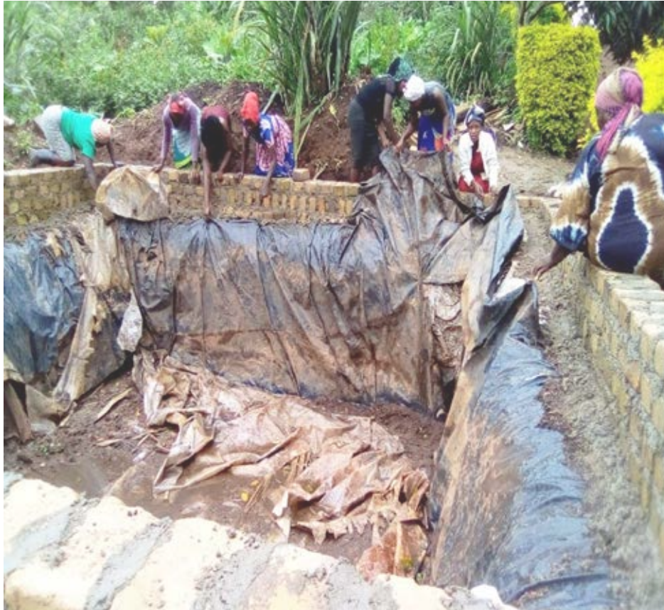
Water pit construction in Uganda SOURCE: St Jude Family Project
